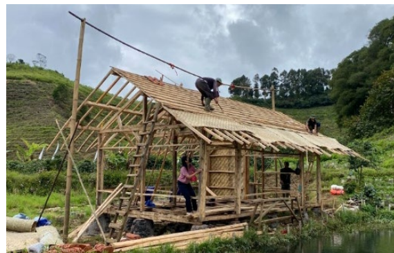
Figure 6. Construction process of the wooden guest house (Pranata et al., 2022).
