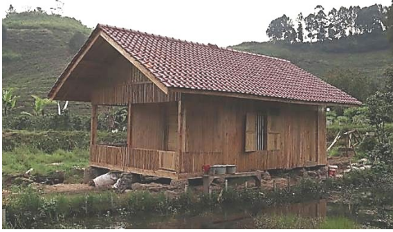
Figure 7. The wooden guest house after completion (Pranata et al. , 2022).
